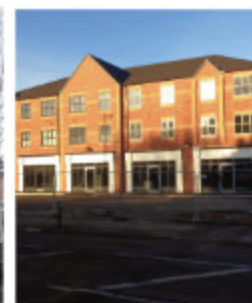
The site of the former Tadcaster Arms. Recently been demolished and the site currently being developed for shops and flats.
